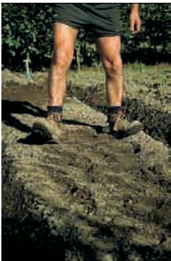
Compacting soil removes any air pockets.
